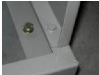
Figure 26 – Floor fixing example
