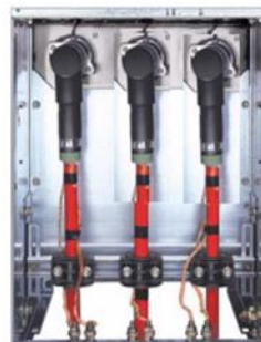
Figure 28 - Examples of Supports and Separable connectors installation
